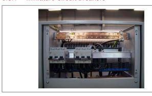
The standard AC output distribution unit is designed with a 35 mm DIN rail, MultiClip termination board and N/PE copper terminal bars, and built as a part of the cabinet.
